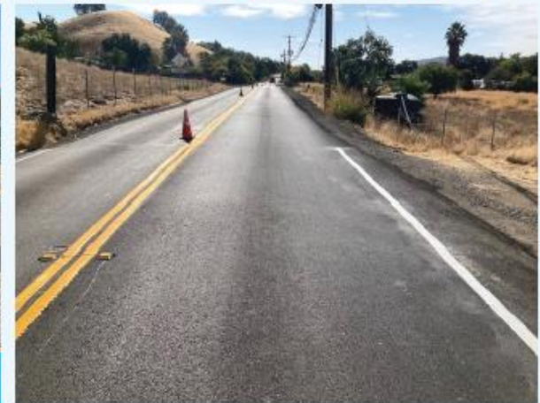
FINAL EDGE-TO-EDGE RESTORATION*
