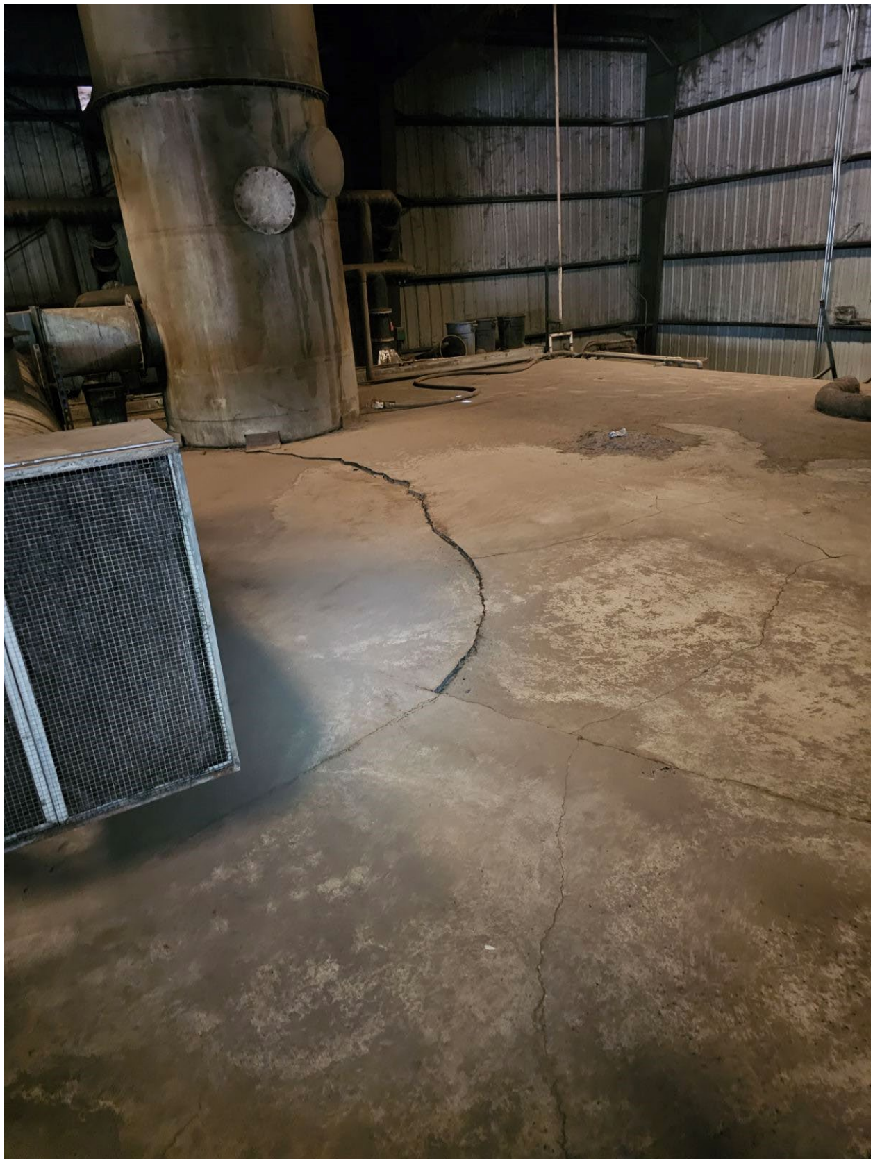
Figure 5: Cracked Roof over Vault #3
