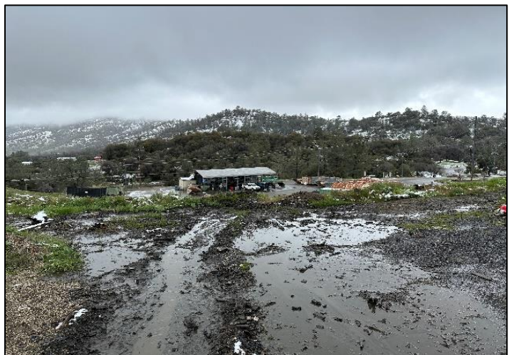
Figure 30 - Poor grading on top of landfill.
