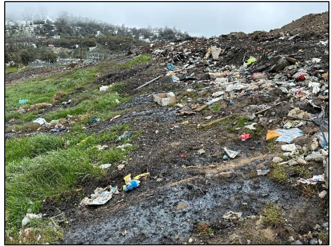
Figure 70 - Exposed waste (not covered) at landfill. Also, some leachate seeps.
