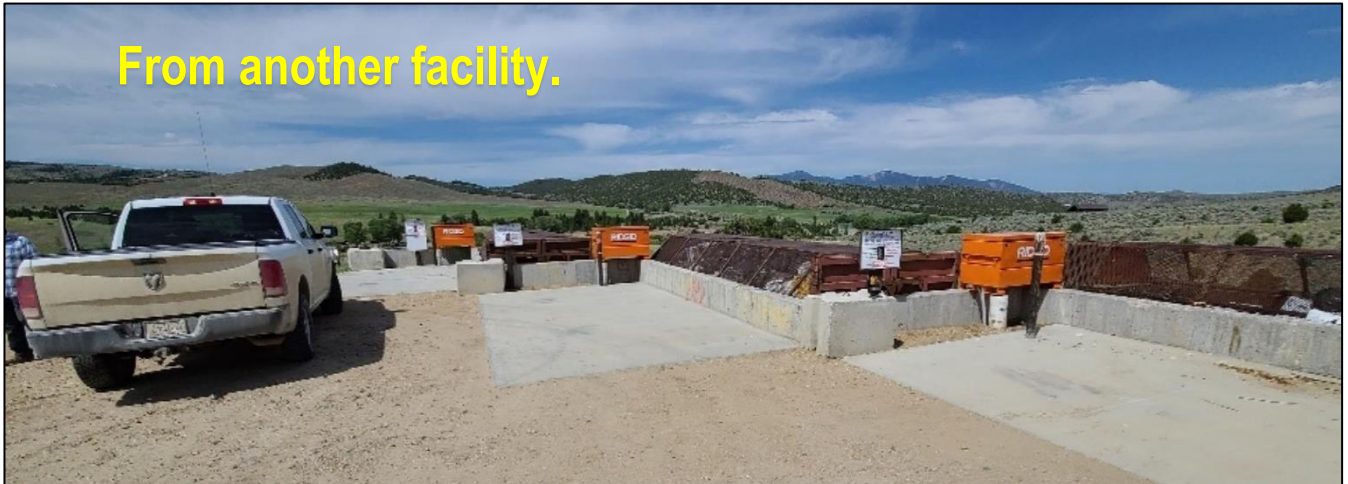
Figure 28 - Hydraulic Lids on Roll-off Containers - Madison County, MT
