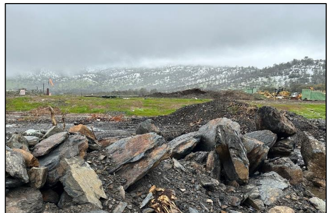
Figure 44 - Oversize slide debris on landfill. Not recommended.
