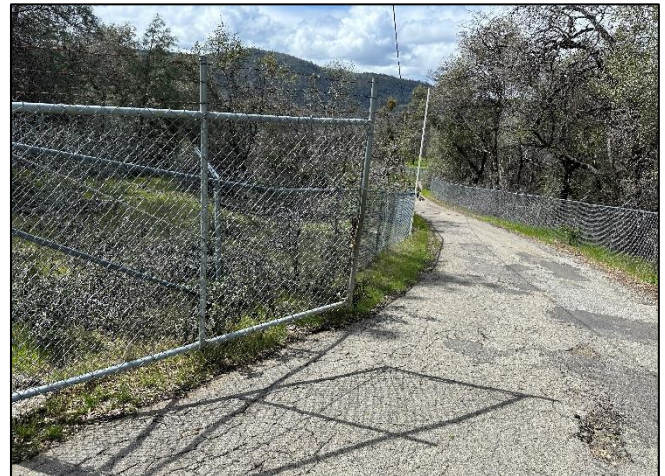
Figure 22 - Coulterville Container Site - Entrance Road
