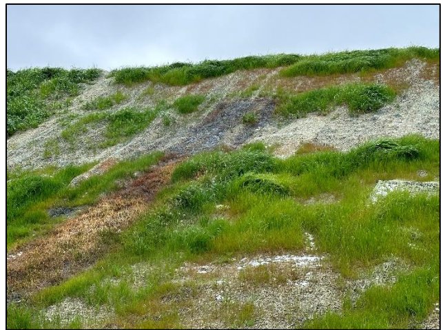
Figure 61 - Leachate seep at mid-slope.
