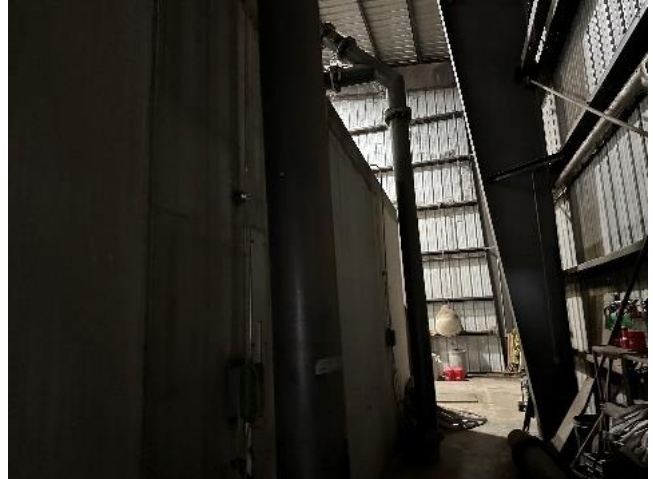
Figure 57 - Piping for the composting system needs to be repaired.
