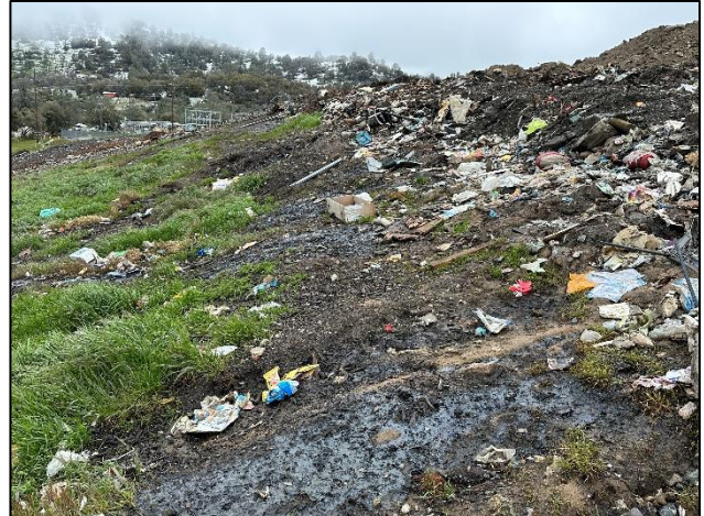
Figure 51 - Area of uncovered waste and leachate seepage.
