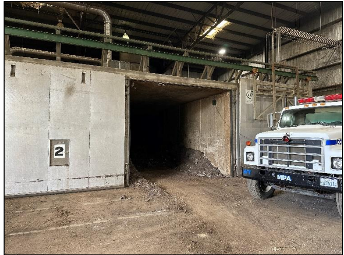
Figure 55- An open bay at Mariposa County's AD composting system.
