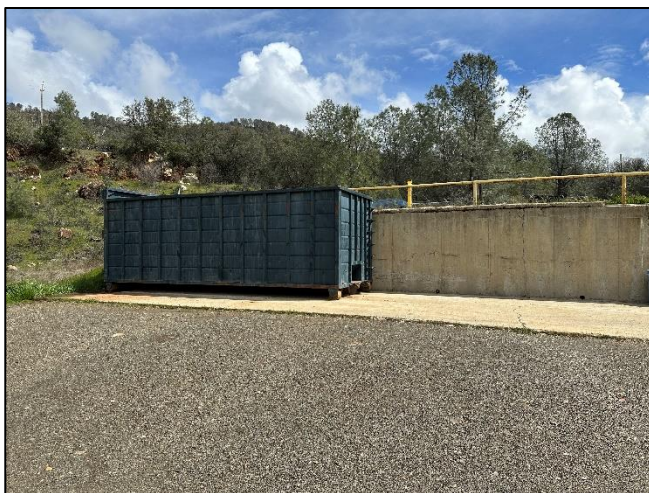
Figure 24 - Coulterville Retaining Wall and Roll-off Bin.
