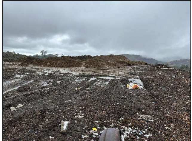
Figure 63 - Ponding causes leachate seeps.
