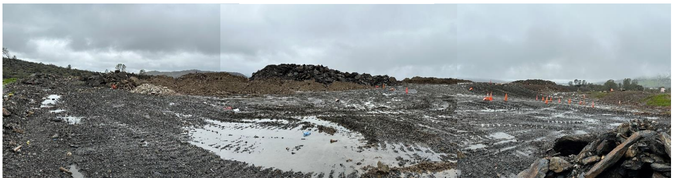
Figure 41 - Ponding on top of landfill.
