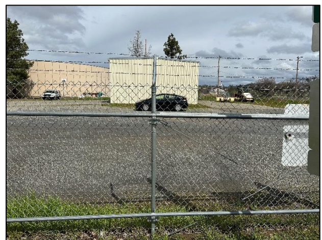
Figure 49 - Good example of site security.
