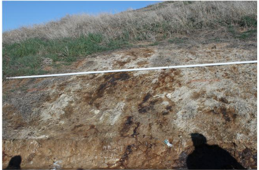
Leachate seeps are a problem for some landfills.
