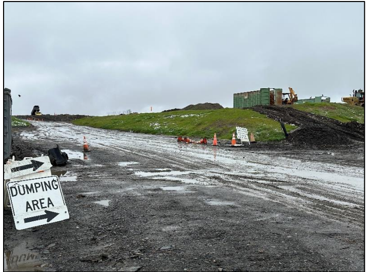
Figure 29 - Access Road to Active Landfill Tipping Pad.
