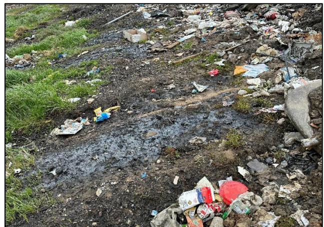
Figure 64 - Leachate seep at top of slope.
