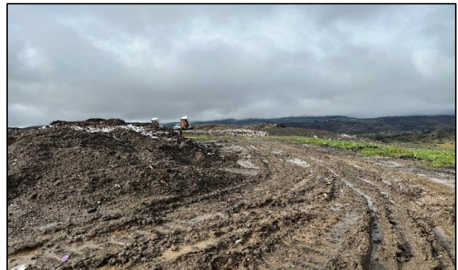
Figure 43 - Muddy, Rutted Access Road.
