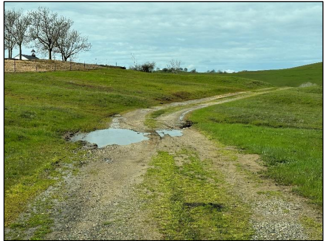
Figure 21 - Hornitos Container Site - Regrade Access Road
