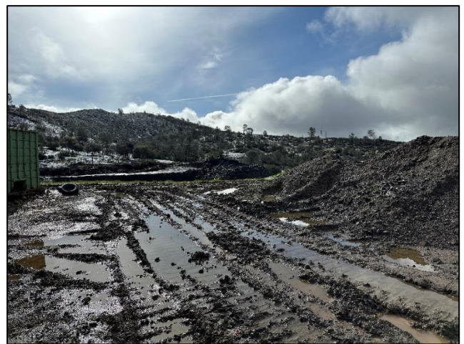
Figure 47 - All access roads should be surfaced for all-weather use.
