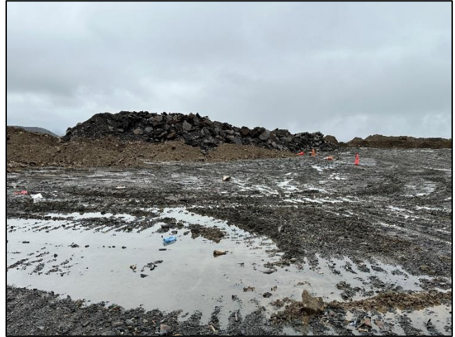
Figure 45 - Stockpile of asphalt debris. Great for road base.
