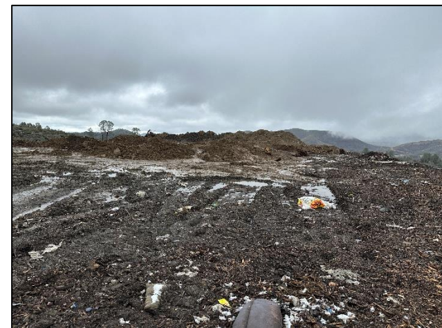
Figure 53 - Poor grading and ponding on top of landfill.
