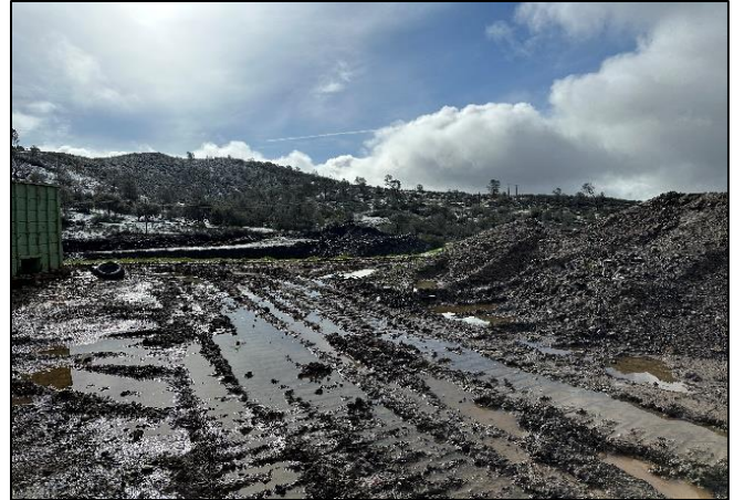
Figure 31 - Poor grading on landfill surface.
