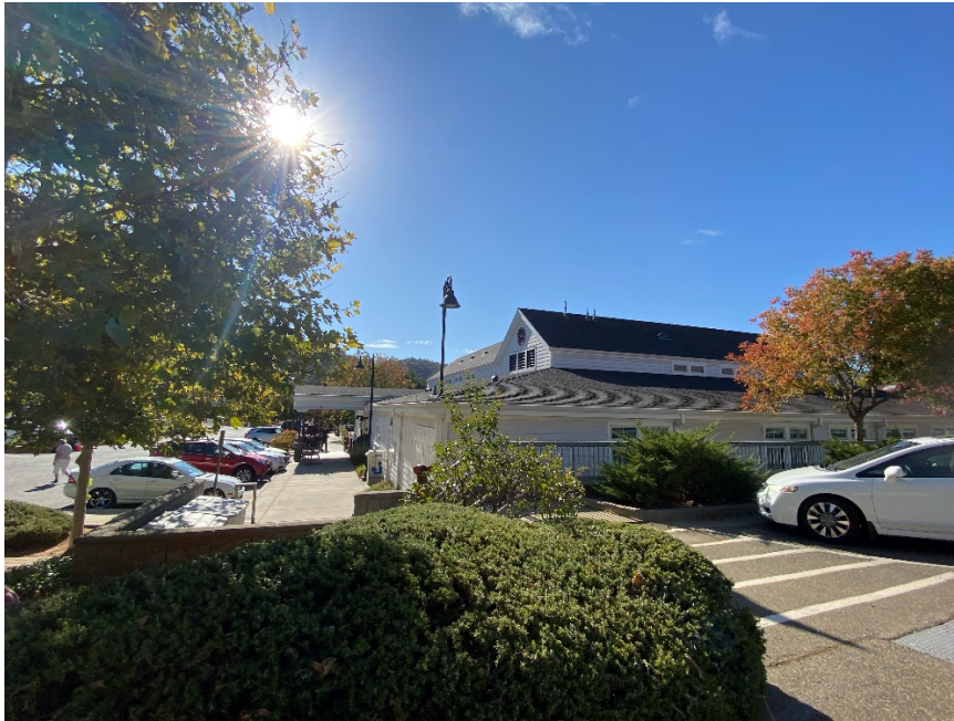
Figure 1 - From Jones Street
