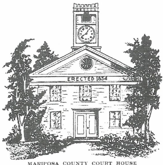
MARIPOSA COUNTY COURT HOUSE
