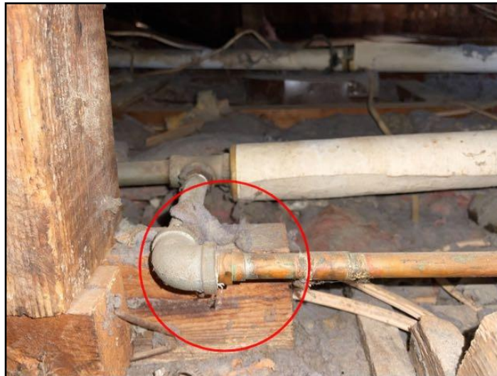
59. Copper/Galvanized Connections
