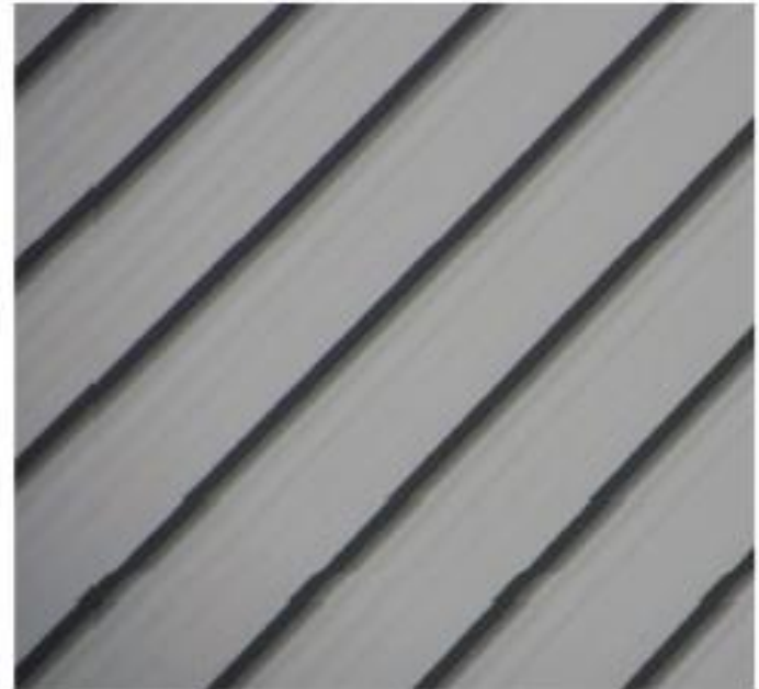
STANDING SEAM METAL ROOFING
