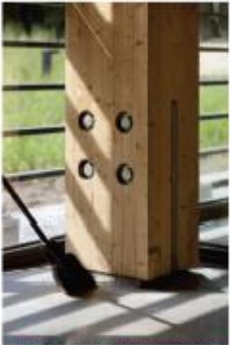
FLITCH PLATE TIMBER FRAMING
