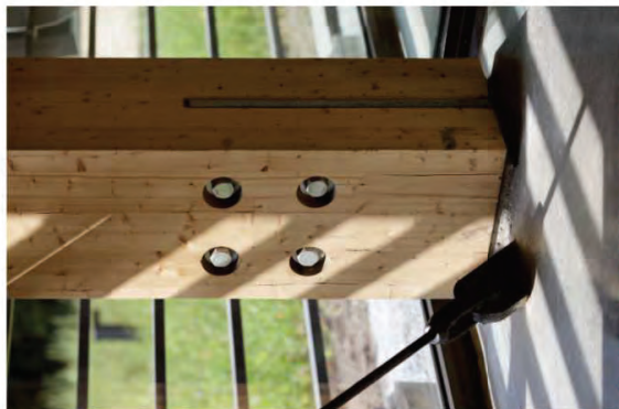
FLITCH PLATE TIMBER FRAMING
