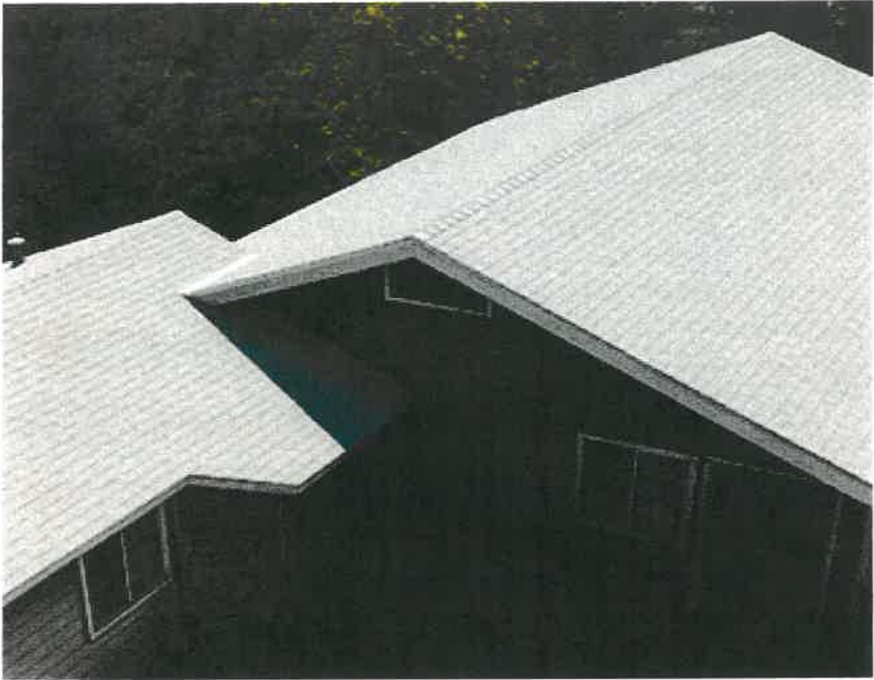
Malarkey dimensional "Legacy" roofing (dove white)
